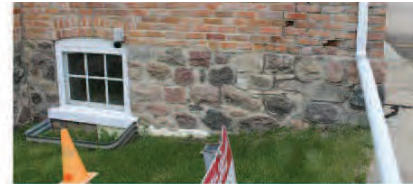
Fig. 49. Severe mortar deterioration at northeast corner of chapel.
