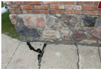
Fig. 50. Mortar deterioration in foundation wall at base of northeast corner of chapel.
