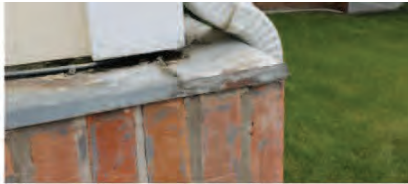
Fig. 48. Back-sloping flashing and gap under second floor siding at northeast chapel corner.
