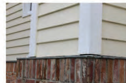
Fig. 54. Typ. paint conditions on exterior siding.
