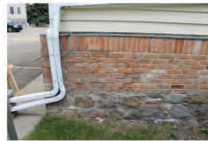
Fig. 51. Mortar deterioration at northwest corner of chapel.
